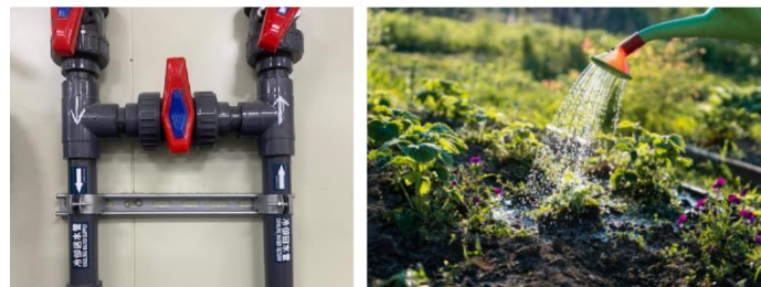
Cooling water recovery system
